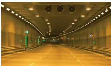
Blick in den fertigen Tunnel
